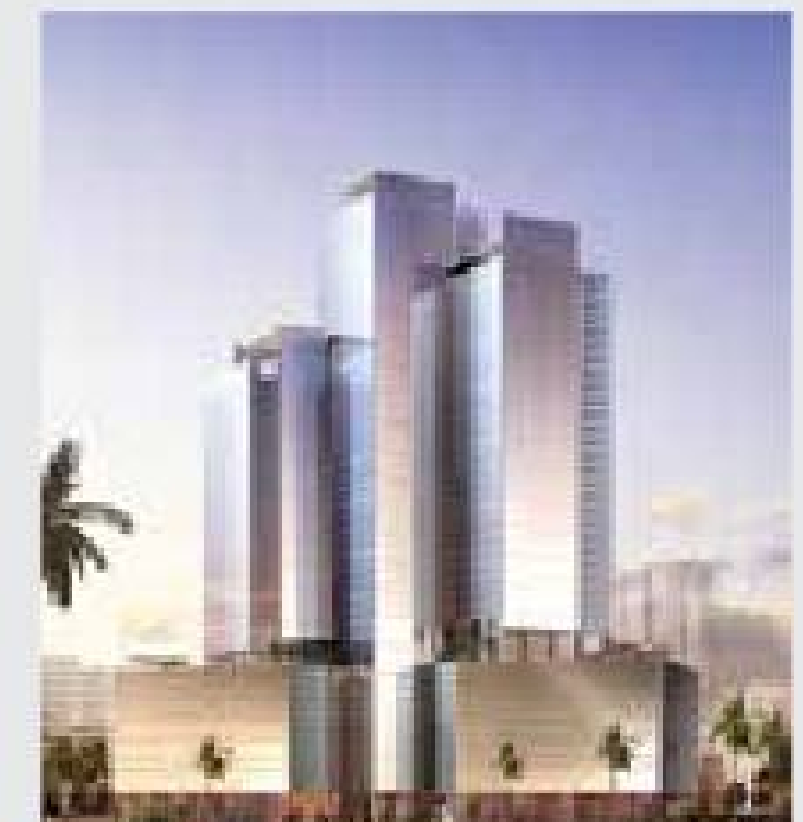
AL SOFFOUH ROAD PROJECT - DUBAI
